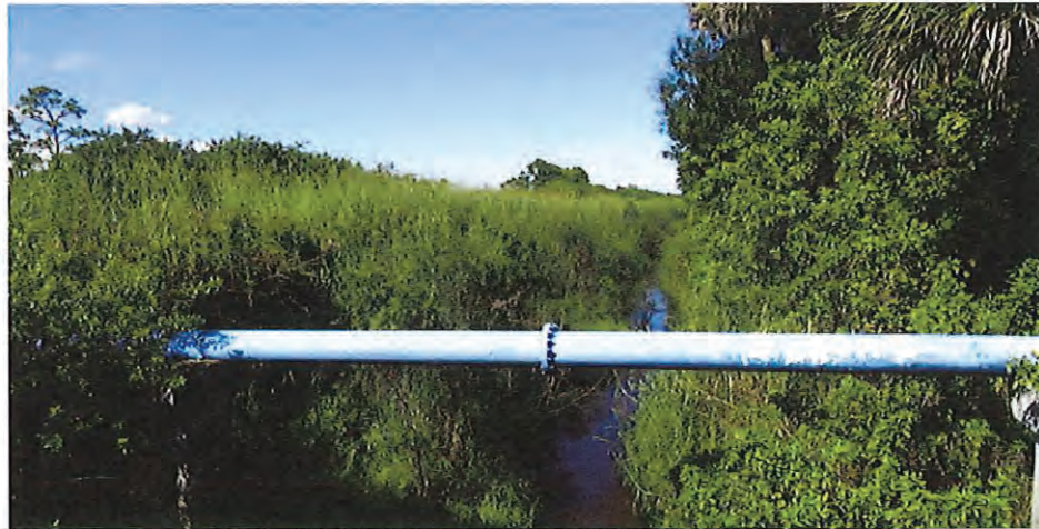
View of drainage ditch along County Road 510
