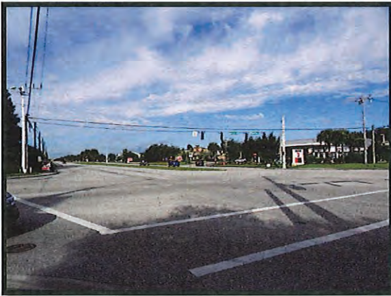
Looking westerly along CR 512 at its intersection with CR 510.
