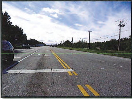
Looking south on CR 510 from its intersection with CR 512.
