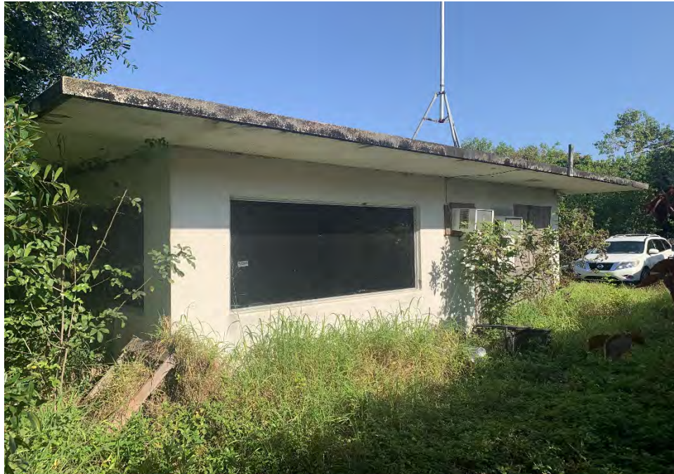
19. View northwest at building improvement not contributing value on actual parent tract and view northwest at TCE Parcel 702 from near its southeast corner. Photo taken 5/15/2025 by Curtis L. Phillips, MAI
