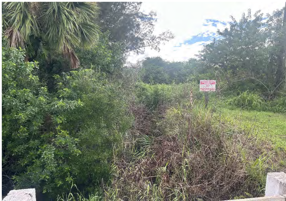
16. View east at typical east-west SRID sub-lateral canal within Parcel 121. Photo taken 9/12/2025 by Curtis L. Phillips, MAI
