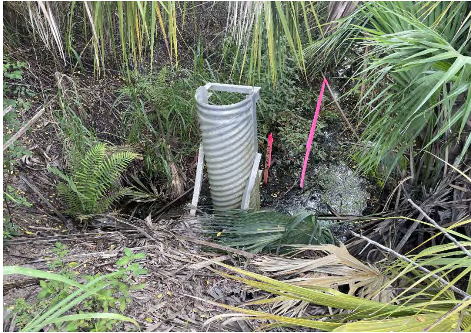
17. View at typical drainage improvements within Parcel 121 that will be replaced by the road contractor.
