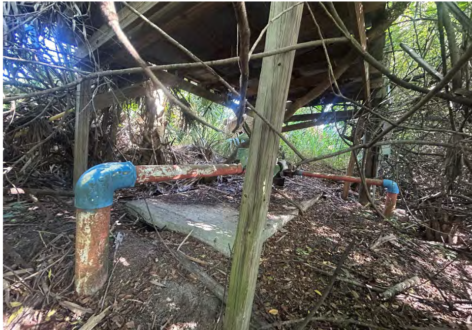
20. View north at shed and piping not contributing value on actual parent tract. Photo taken 7/24/2025 by Curtis L. Phillips, MAI
