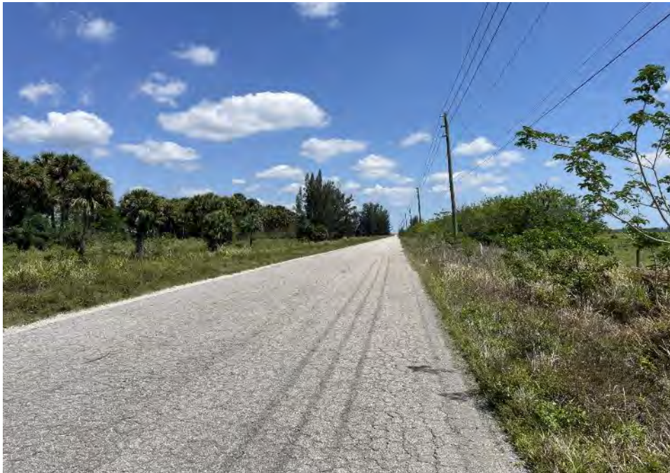
2. View north along 82 nd Avenue. Photo taken 5/15/2025 by Curtis L. Phillips, MAI
